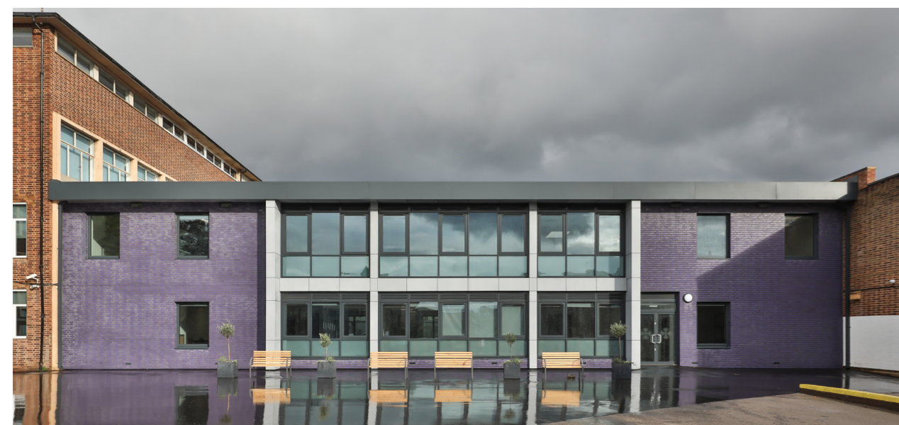
Existing 'Rome' Building
