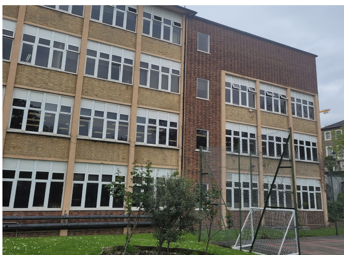
Existing Site Photograph - Existing Facade Condition
